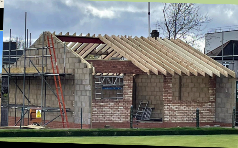
The roof takes shape
