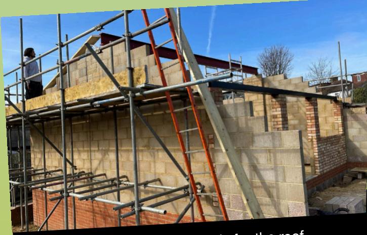
The scaffolding is in place ready for the roof
