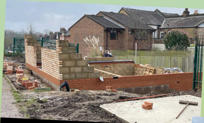
The walls start to go up
