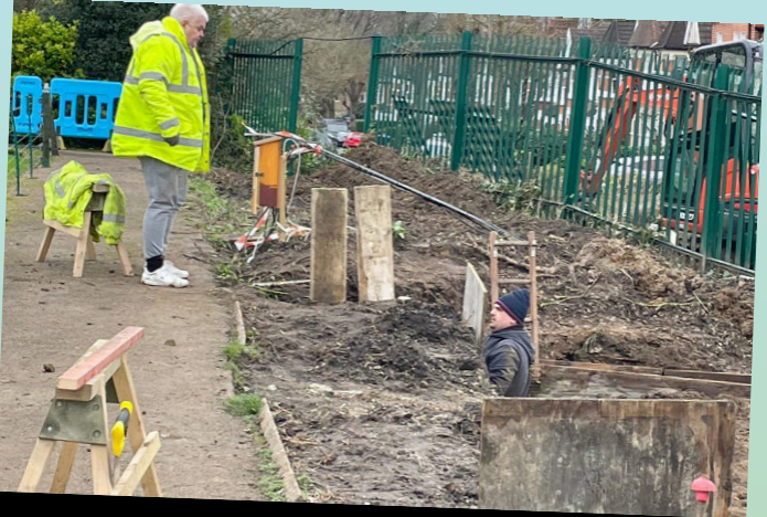
The foundations were dug, but the council came along and said they had to be deeper. These are the finished depth, note the man in the hat standing in them for scale.
